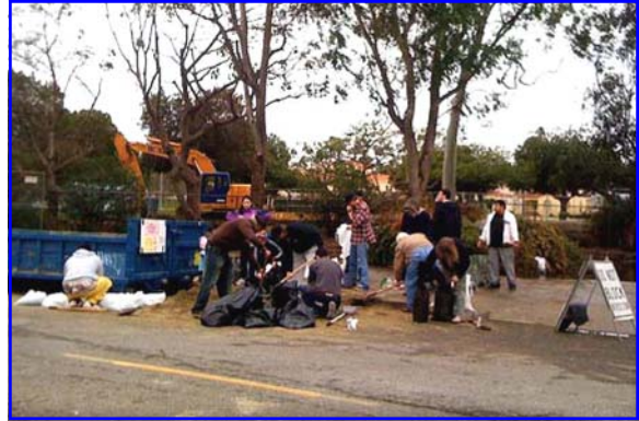
Sandbagging at Station 14
