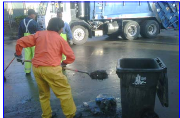
Crews Clean Up
